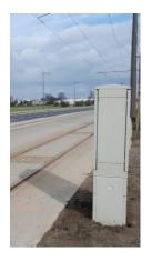
An industrial enclosure or street cabinet contains the data acquisition module and an industrial computing unit. The box is installed in the vicinity of the track up to a distance of 150 m.
