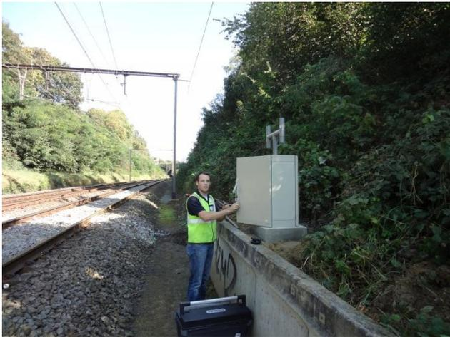
The APT-WIM system (Weigh In Motion) is specifically developed for the determination of the dynamic load impact from the vehicle on the track.
