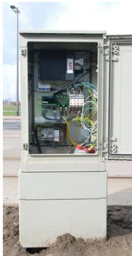
An industrial enclosure or a street cabinet contains the data acquisition module and an industrial computing unit. The box is installed in the vicinity of the track up to a distance of 150 m.
