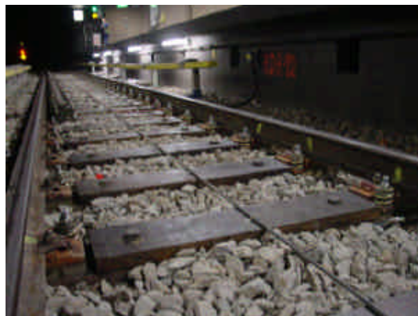
Figure 6: Detail of the very resilient fastening system
