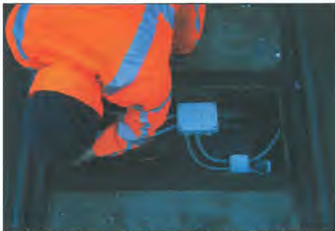
Fig. 1: APT-WORM equipment being installed in an embedded track
