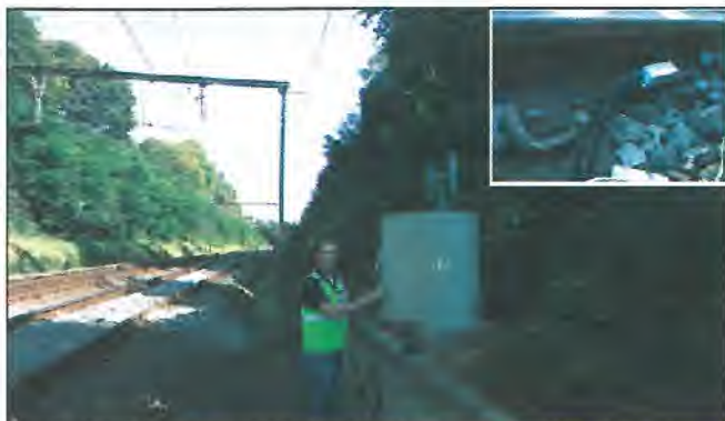
Fig. 2: APT-WORM sensors installed on ballasted track
